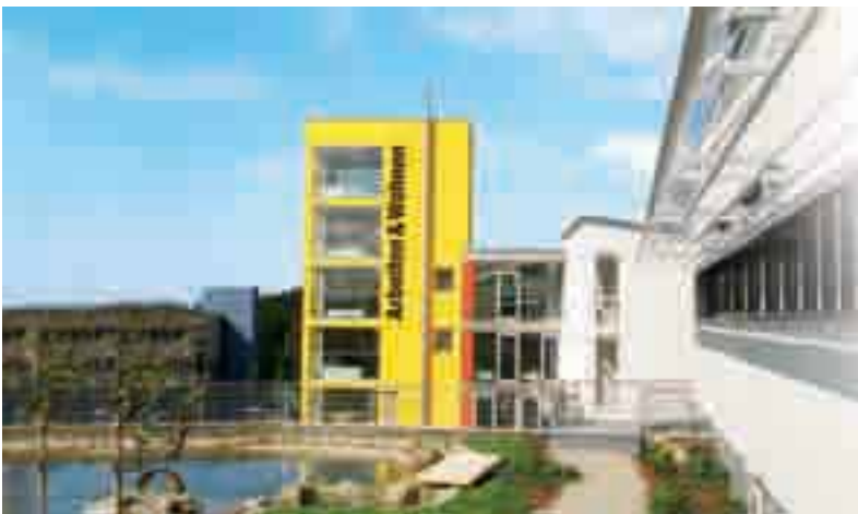
The newly completed "Living & Working" building, which offers offices and home accommodation to company founders.
